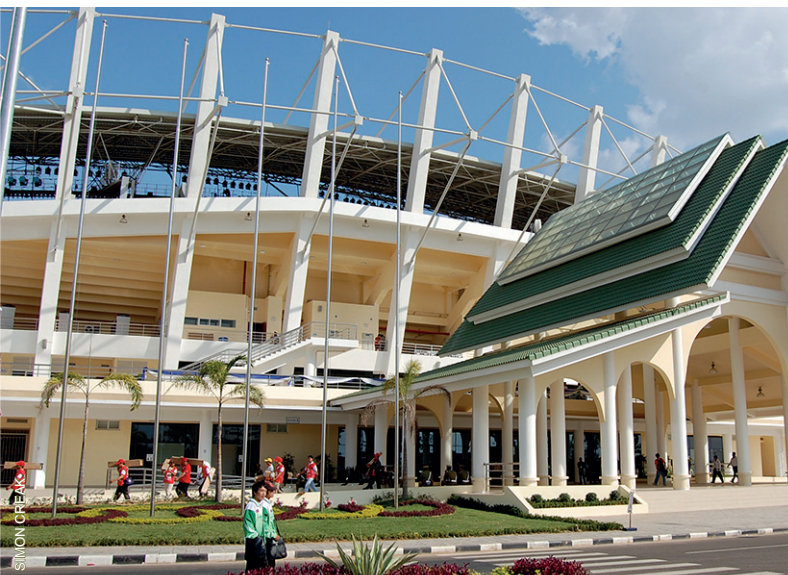
Fig. 7 (below right). Entrance to the US$19m SEA Games Village, funded by a Vietnamese company, reportedly in return for logging concessions and a hotel deal.
